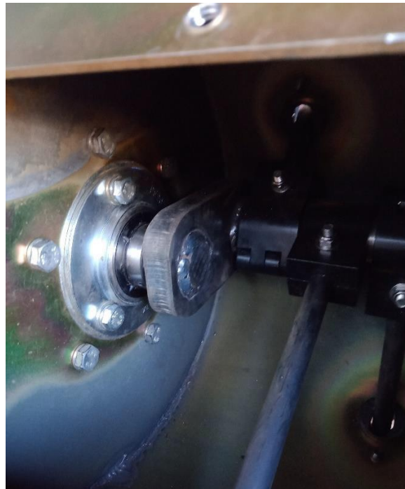
Figure 7: Bearing at the drive end, when looking from the inspection slot
